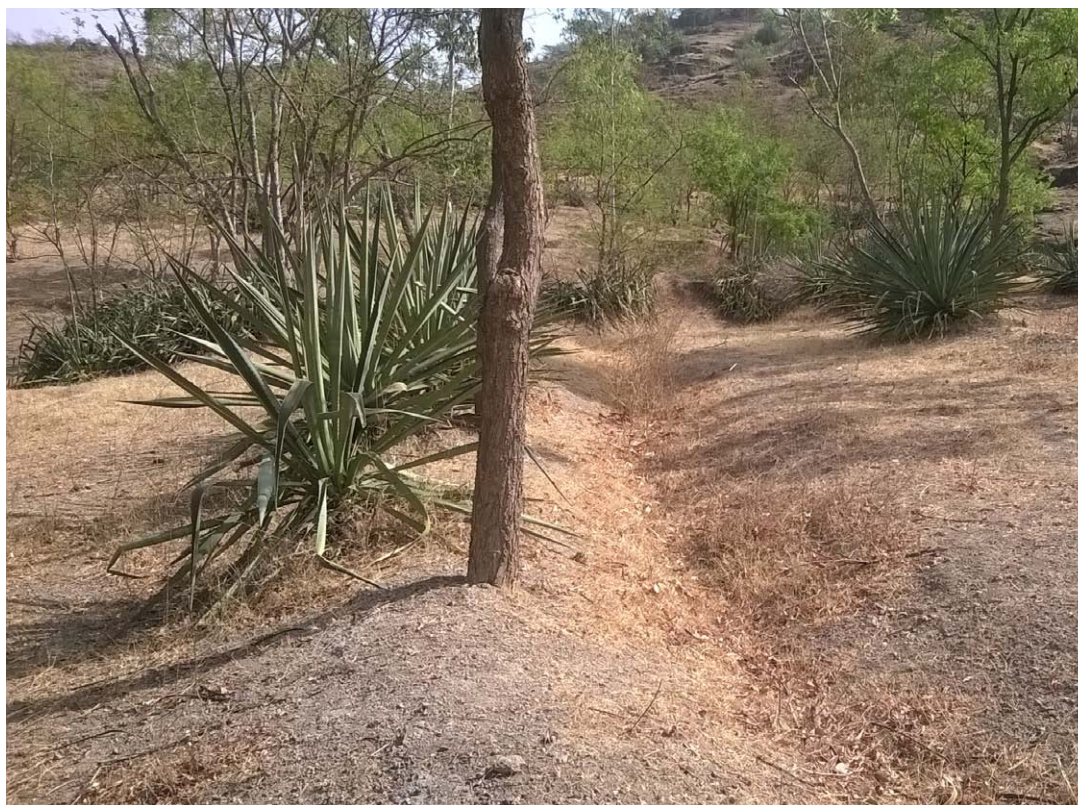
Contour trench in common area during the dry season in IGWDP intervention region in India © S. Srigiri
