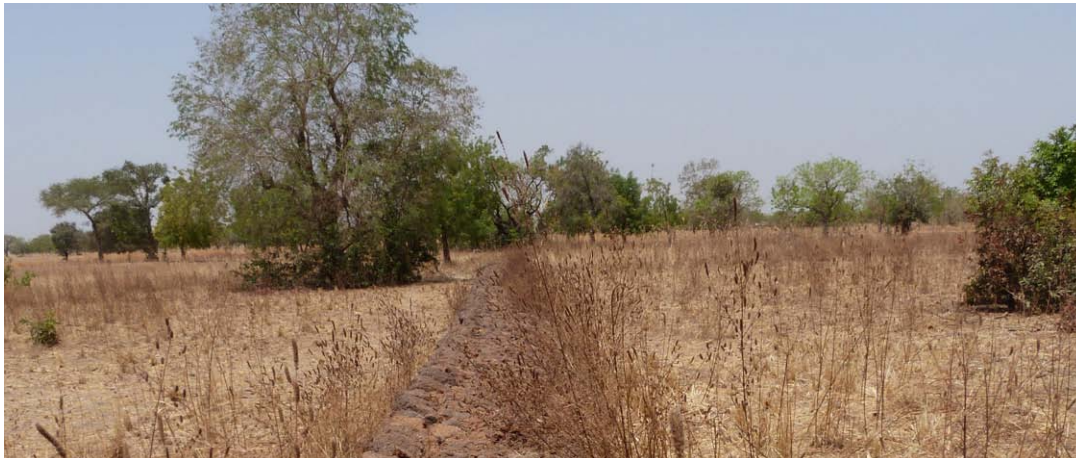
Stone bunds delimiting field in Mouyoupin village (Burkina Faso) EKF Programme ©T. Jenisch
