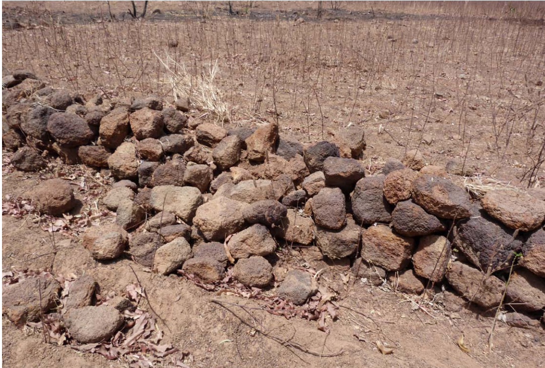
Lack of maintenance of a stone bund in Koumbia village, Burkina Faso ©T. Jenisch
