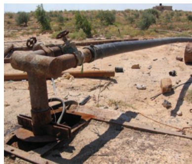
Figure 4. Illegal well in Azraq: no meter is installed.
