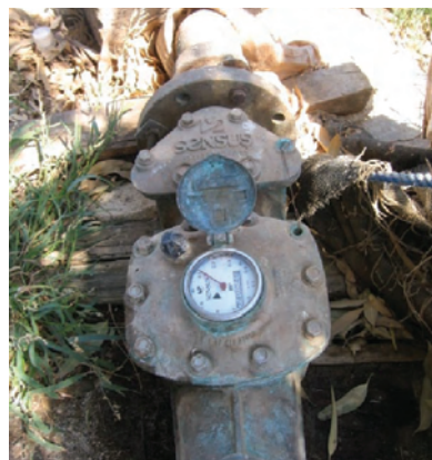
Figure 5. Meters installed on legal wells are used to calculate water consumption.
