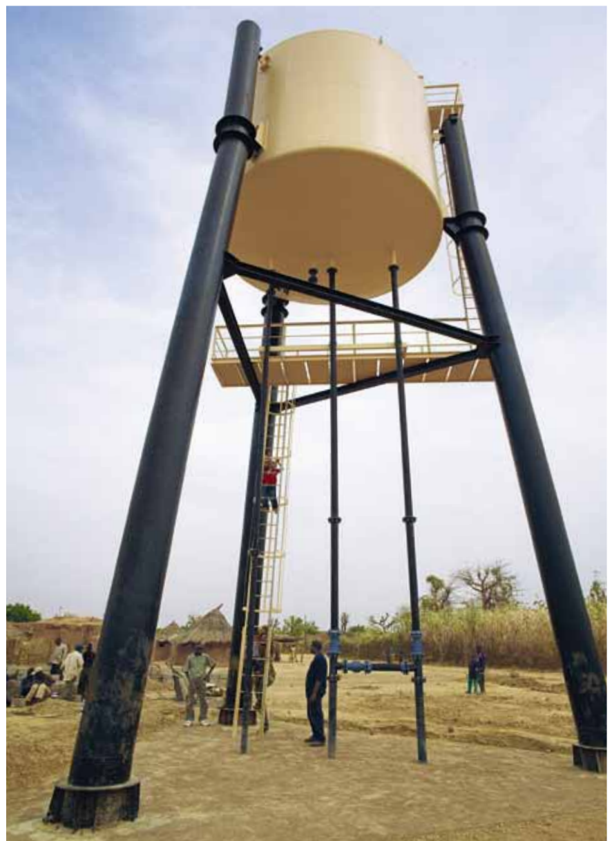
Deep wells are becoming increasingly important in the Sahel Zone.
