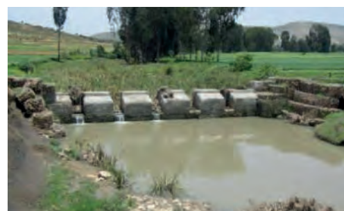
Check dam made of stone, concrete and gabion for irrigation purpose at the same time reducing the runoff velocity and enhancing gully rehabilitation. (E. Yazew)
