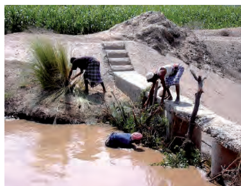
Blocking scour sluice on a modernised spate irrigation system in Yemen. (spate-irrigation.org)
