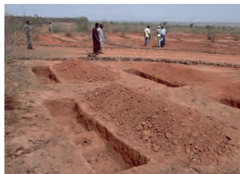
Microcatchments for tree planting, Ethiopia. (HP. Liniger)
