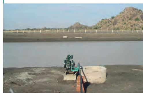
Excavated pond (improved hafir system) with water pump and sedimentation tank. (Ministries of Water Resources and Irrigation of Sudan and South Sudan, 2009)
