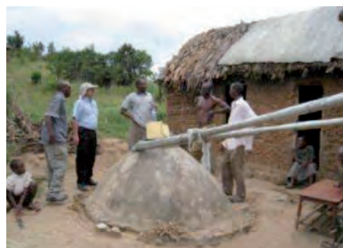
Organic roof with an additional plastic covering and partially below ground tanks in rural Uganda (Danert and Motts, 2009).
