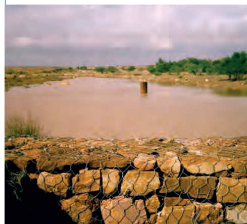
Example of a recharge well behind a gabion check dam after rain. (M. Ouessar).
