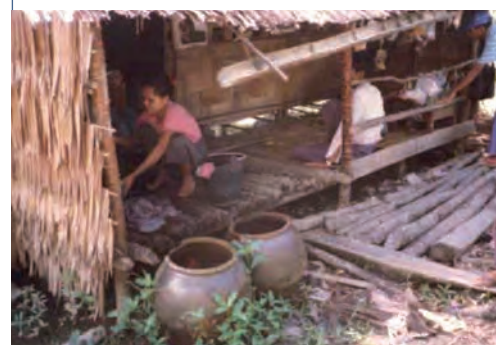
For more permanent guttering bamboo is split, tied to a few sticks and fastened with a gradient to the rafter of the house.
