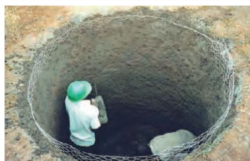
Underground tank for courtyard and road water harvesting, Kenya. This tank was equipped with a silt trap and used for storing runoff (Nissen-Petersen, 2007).
