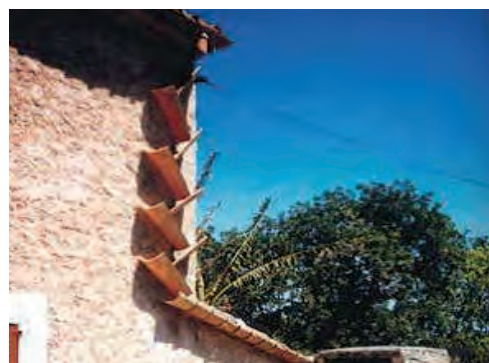
"Cascading gutters" of a RooftopWH system for domestic use in Mallorca, Spain (Barron, 2009).
