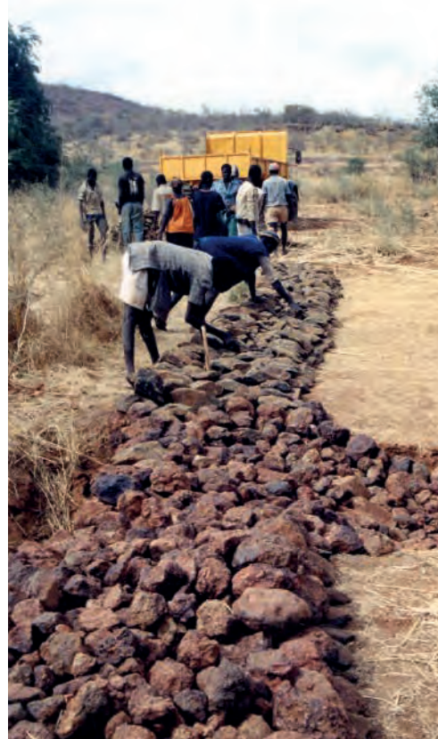
Constructing a permeable rock dam ( digue filtrante ) in Burkina Faso. (W. Critchley)
