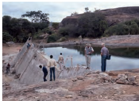
Construction of a rock catchment dam in Kitui, Kenya. (HP. Liniger)
