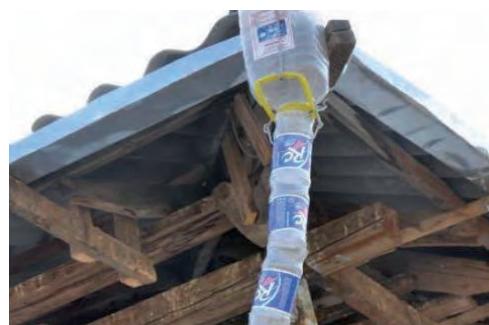
A fallpipe made of old plastic bottles stitched together by thin wire, Tajikistan. (S. Stevenson)
