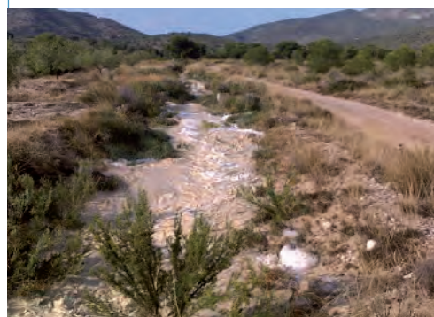
Traditional channel system ( acequia ) directing diverted flood water (by earthen or stone bunds) from intermittent streams towards almond terraces, Spain. (J. de Vente)
