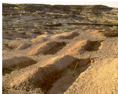
Microbasins or trenches ( tranchées ) in Niger. (HP. Liniger)
