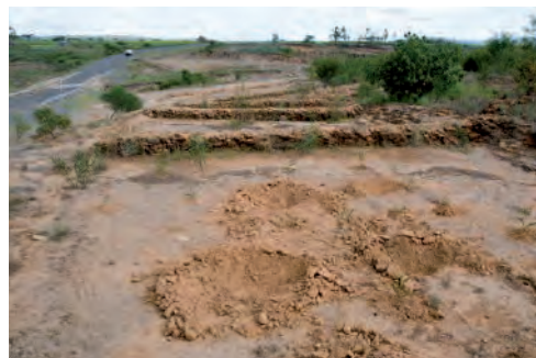
Road runoff harvesting system with macro- and microcatchments in Ethiopia. (HP. Liniger)
