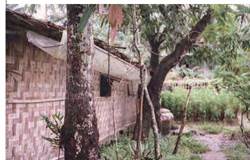
When rain is expected the house owner attaches a wide and removable gutter made of plastic sheet below the roof.
