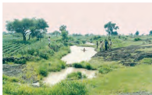
A series of dohs temporarily filled with runoff water before infiltration. (D. Gandhi)
