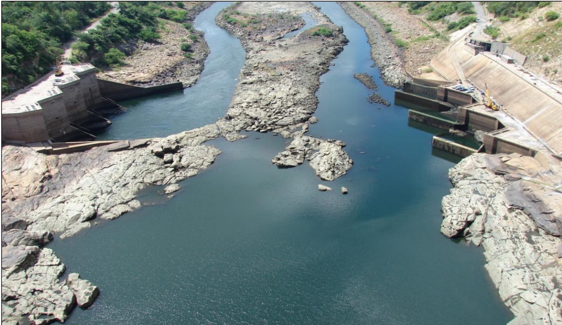
Figure 5.1: Kariba Dam Power Stations' Tailrace Outfalls
