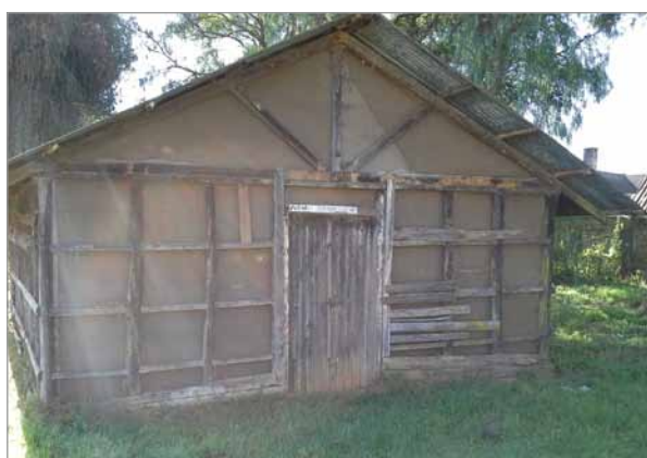
Photograph 3: Seed potato storage - diffused light store
