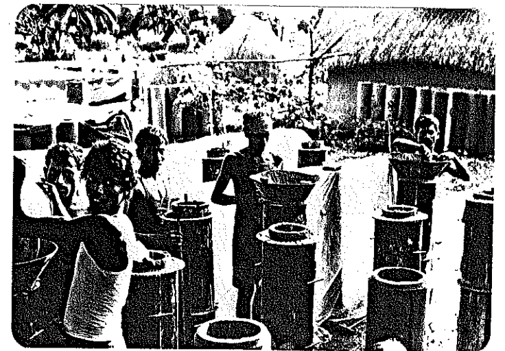
CC Pipe casting in vertical moulds
