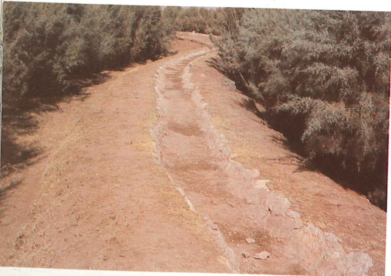
A feeder channel equipped with concrete, with shelter belts on both sides.
