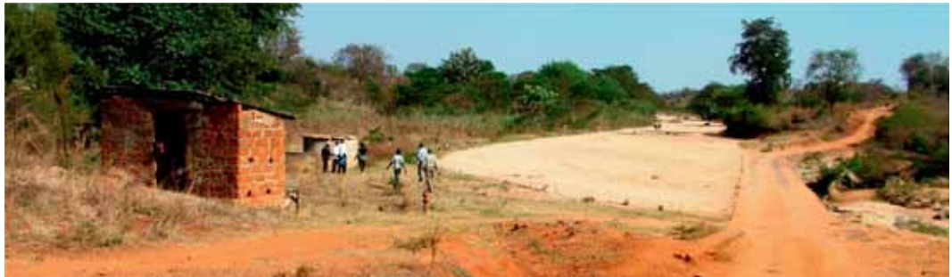
A double sand dam used as a rural road in Machakos County, Kenya. An infiltration gallery is connected to a shallow well and a pump. This dam crossing yields an estimated 40 million litres of water per year.
