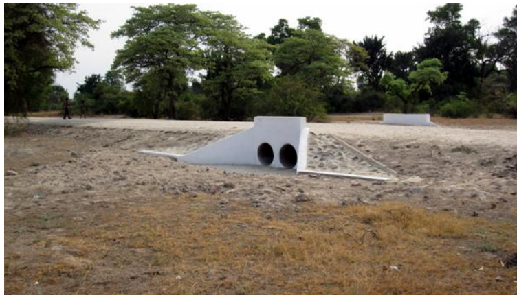
Figure 7.1: Recently improved roads and culverts in Caprivi strip (photo visit October 2010)
