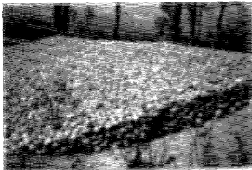
Protected dyke through forest belt, Udayapur; when sizes of locally available stones are small, thickness of boulder work should be increased
