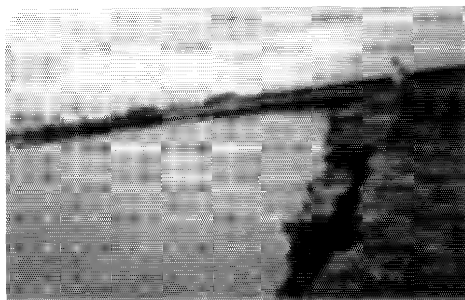
Slumping of bank during high flood.
