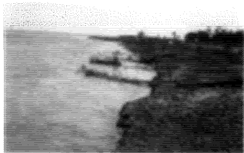
Bamboo pile spur for bank protection during flood situation.
