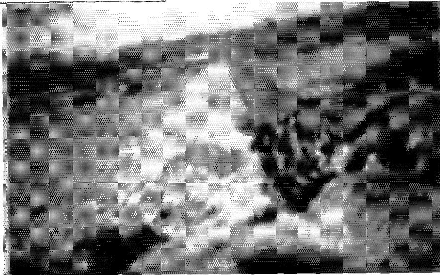
Toe and slope protection work of an earthen embankment by dry boulder pitching and plantation
