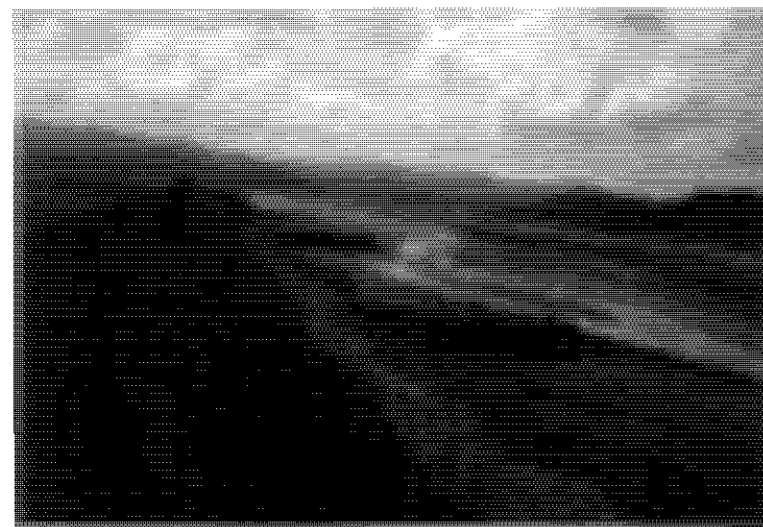
Sediment deposition between the spurs establishing the embankment.
