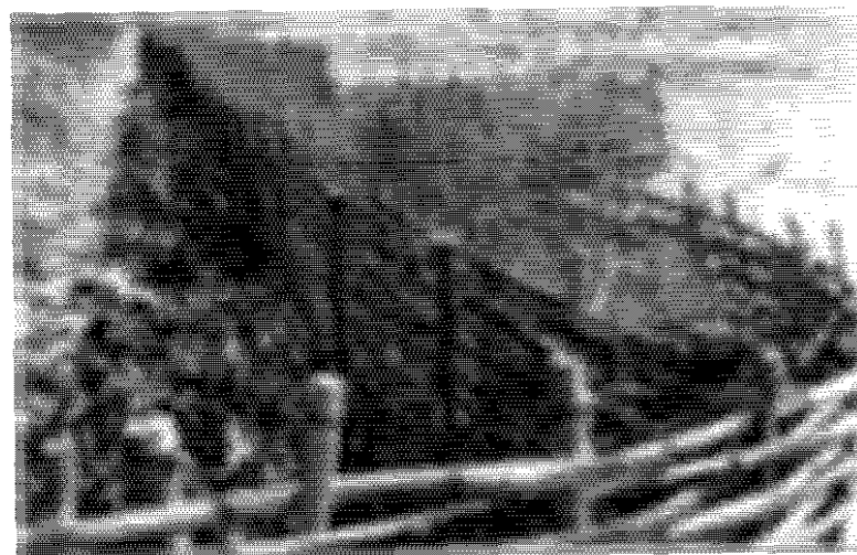
Protection of an earthen embankment by bamboo piling and plantation.
