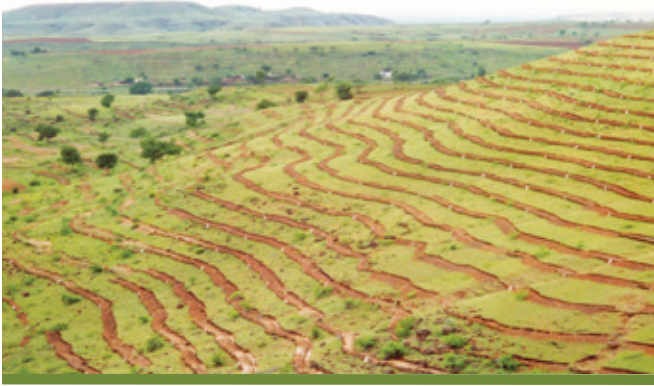
Contour trenching for runoff collection
